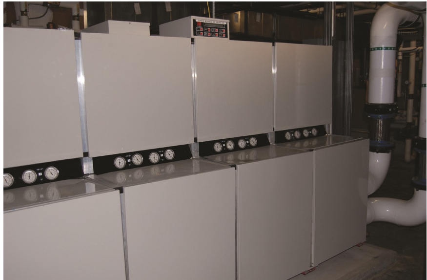
The 200-ton modular scroll-chiller system at Proximity Hotel.
